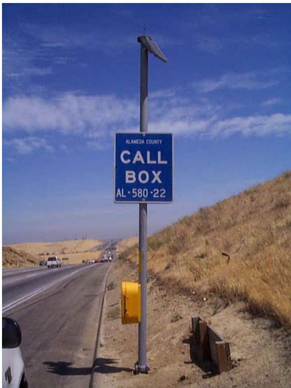
Site Type L – installed behind a curb.
