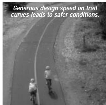
*Use a realistic design speed on separate trails.* Twenty miles per hour is a reasonable design speed on level ground. On hills, increase it to 30mph or more.
