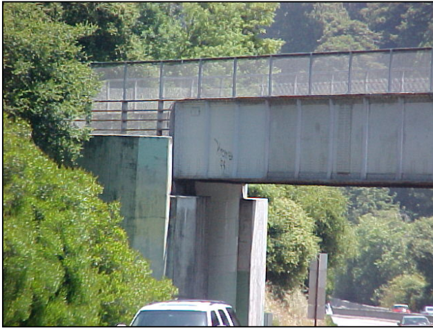
Abutment 1 Looking D/S
