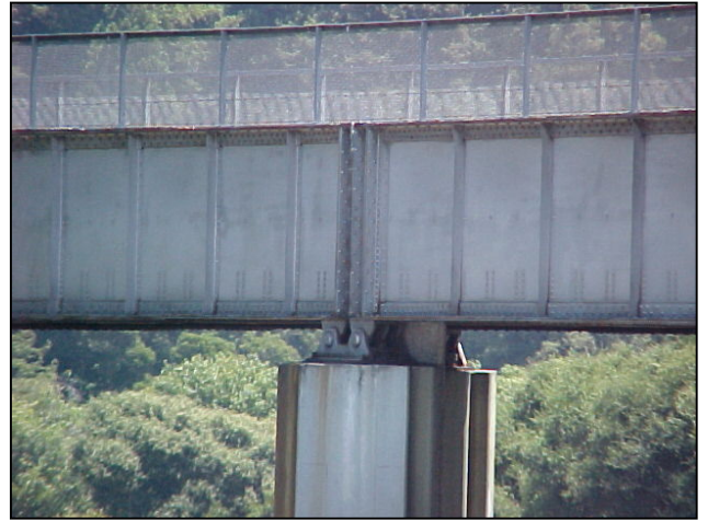
Bent - Girder Connection
