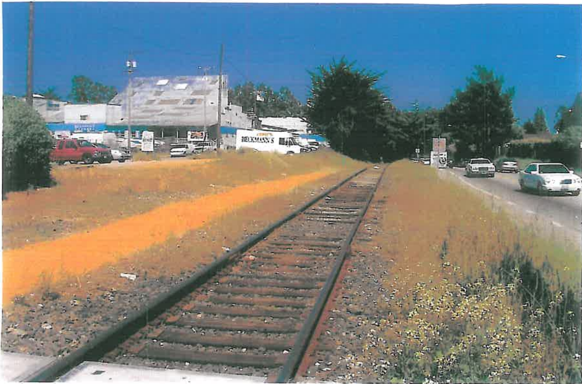
RR looking east from Seabright Ave (City of Santa Cruz)
