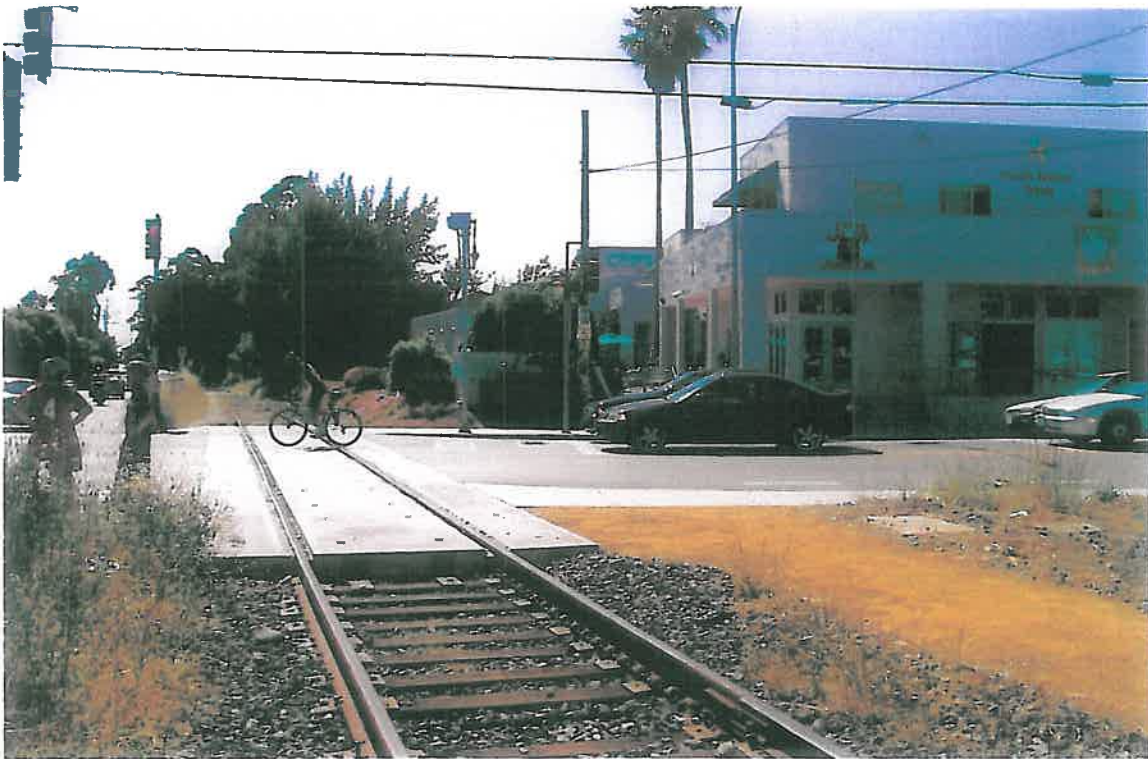
RR looking west across Seabright Ave.
