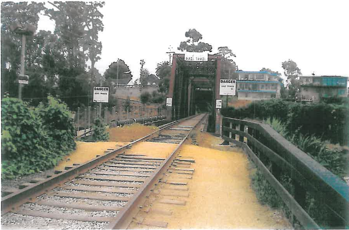
RR trestle across San Lorenzo River looking east from east end of amusement park.
