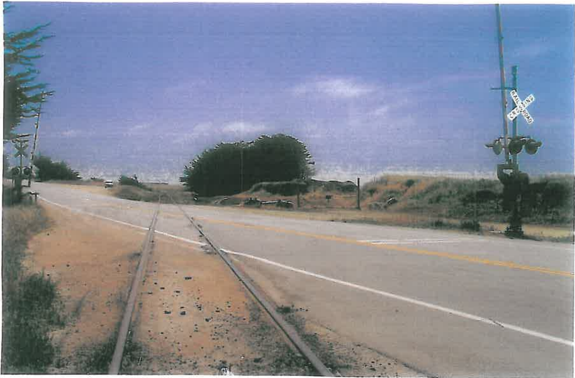
RR looking south across Hwy 1 at cement plant north of Davenport.
