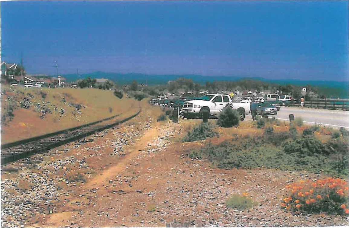
RR looking East from point where Cliff Dr (to right) has houses between it and the shore – Rr is below houses to left and at or near the road grade which is gentle here.
