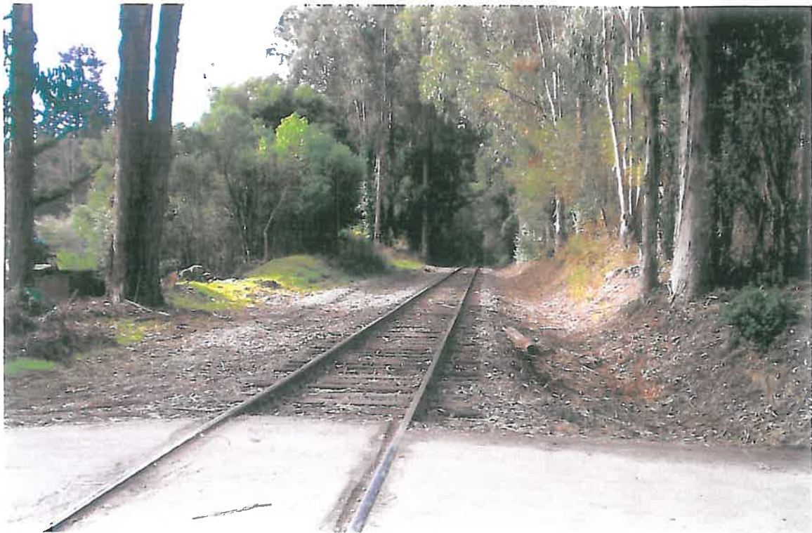
RR looking east from New Brighton Dr. (State Park on both sides – New Brighton Dr.)
