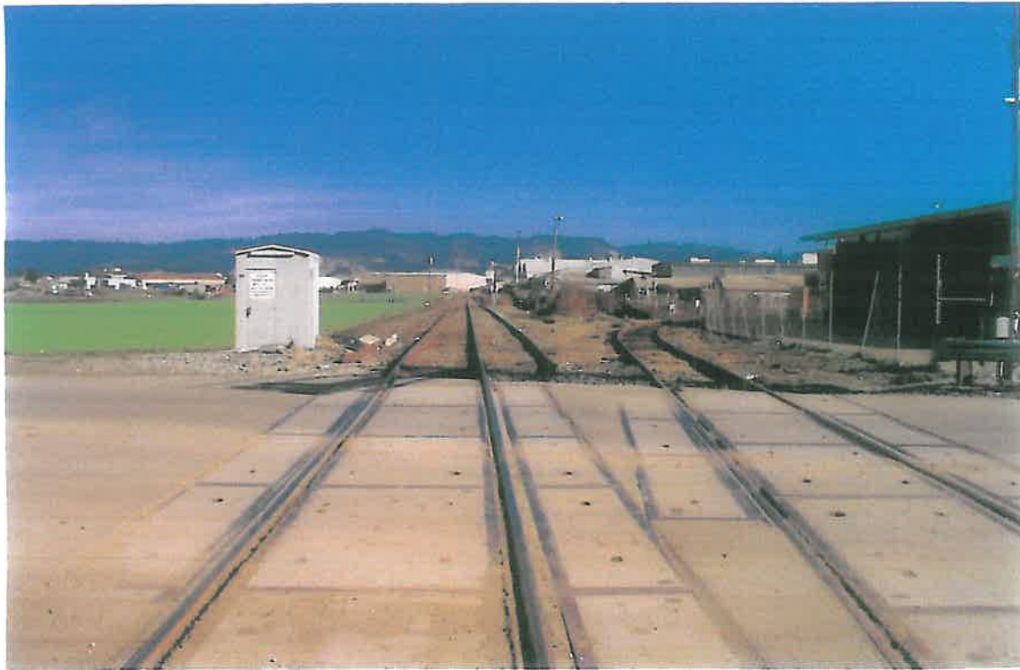
RR looking E across Errington Rd (spur to right leads to system of spur tracks on easements – not part of the sale). Watsonville City limits on L side of R/W; county agr. To Left, county industrial uses to Right
