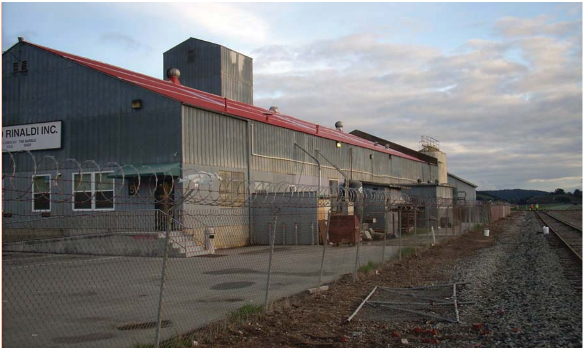
Photograph 1. Gino Rinaldi, Inc. property. Approximate milepost 0.7. View to south-southeast along the Branch Line.
