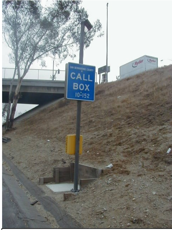
Site Type B – installed in a cut-slope.
