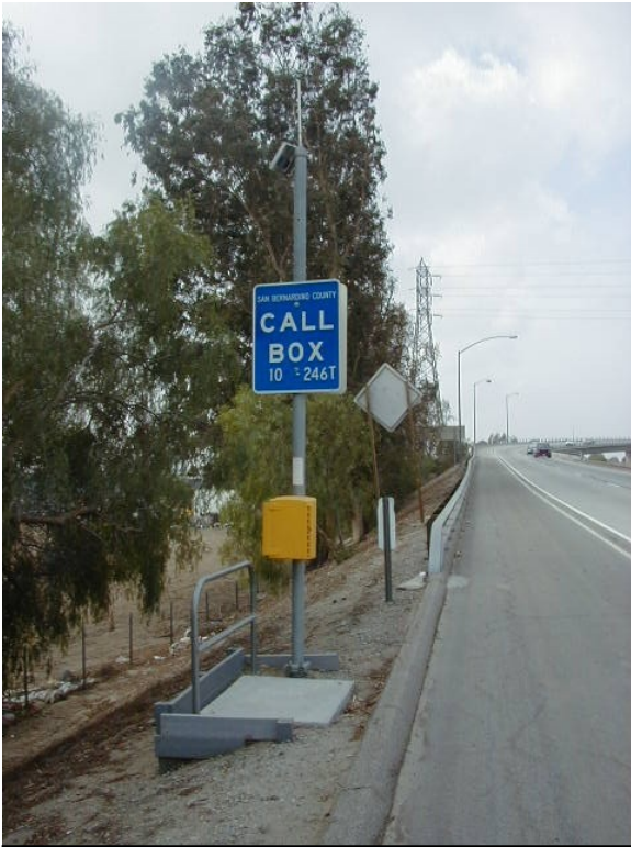
Site Type C – installed on an in-fill slope.
