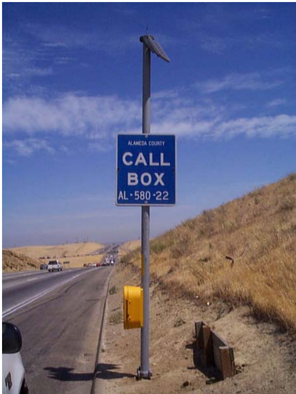
Site Type L – installed behind a curb.
