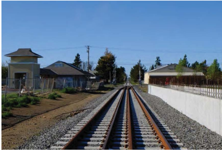
Gantlet track (additional set of rails) adjacent to high level platform (under construction) at the SMART project.
