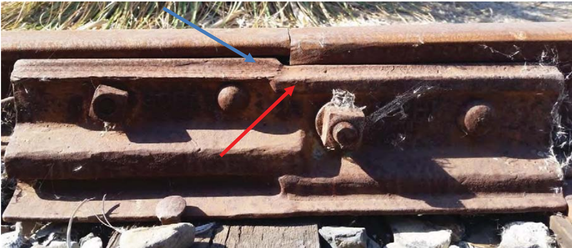
Figure 6-1: Joint Bar
