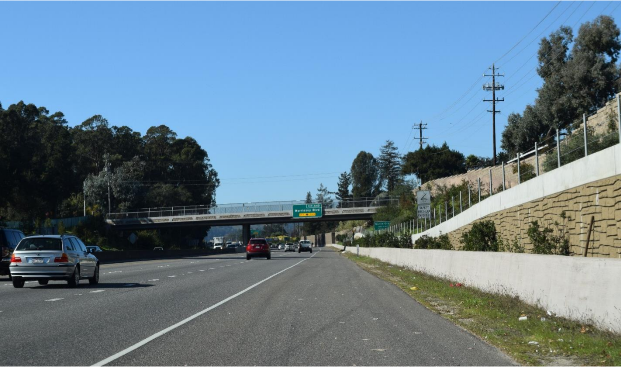
Figure A: Typical Viewpoint 23, before the Auxiliary Lane Project (top) and after (bottom).
