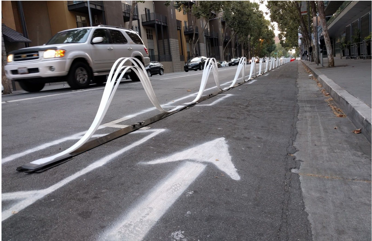
Pop-up protected bike lane in City of San Jose - Photo credit: City of San Jose
