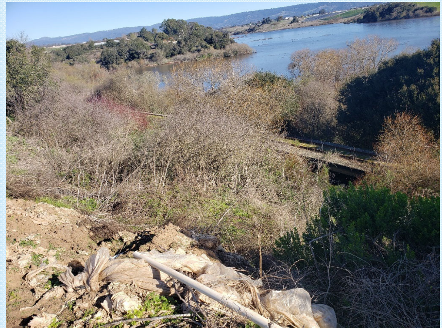
View of Bridge from Agricultural Field, looking east
