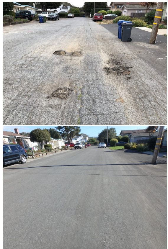
Measure D-funded road resurfacing – Santa Cruz Avenue, Seacliff Beach - Before & after
