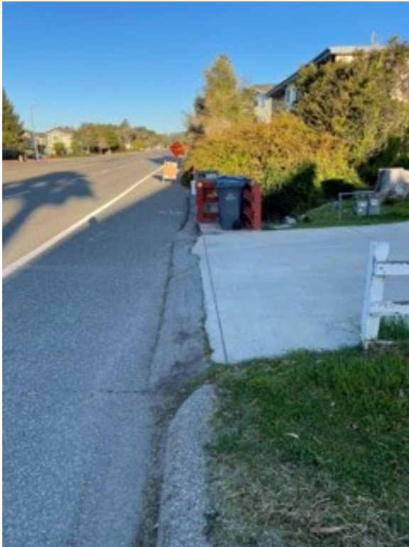
Lack of sidewalks along Soquel Drive
