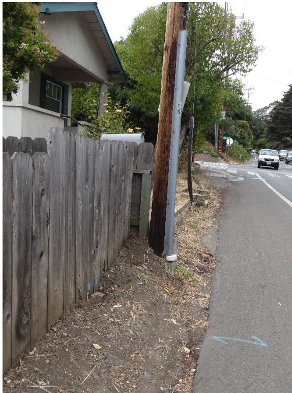
Lack of sidewalks
