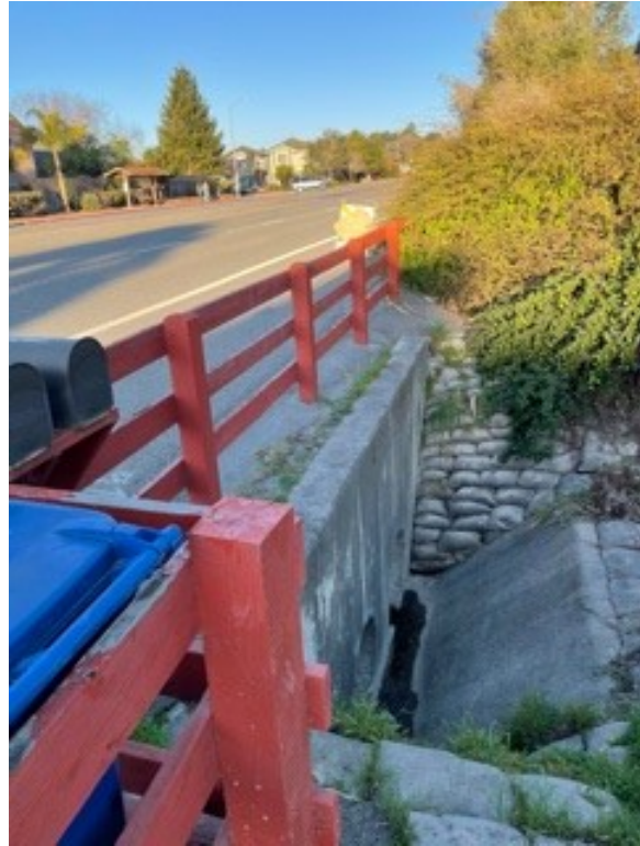
Retaining wall and fencing
