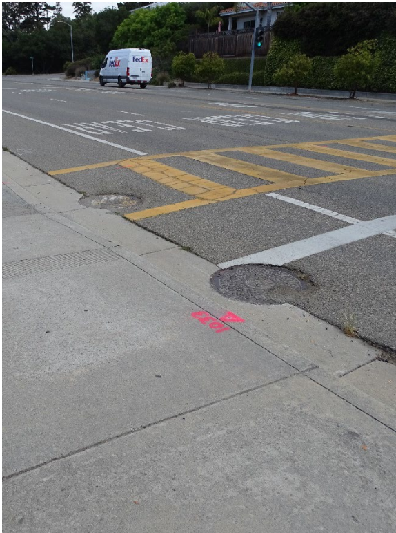
Existing midblock crossing to be upgrade
