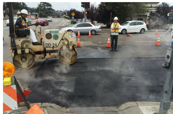
Paving at State Park Drive
