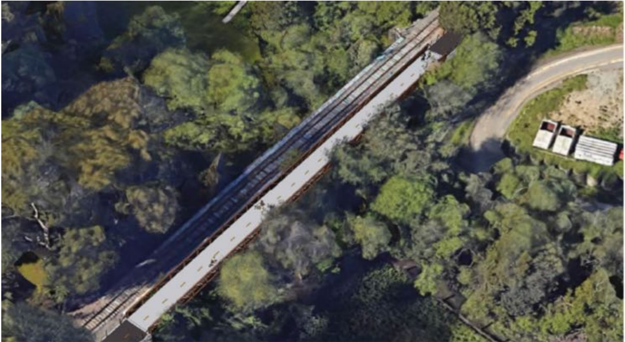
Rodeo Gulch clear span bridge.
