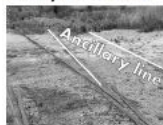
Ancillary line lost in dirt
