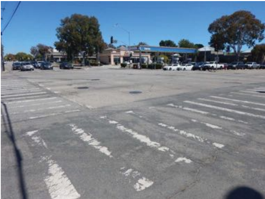
WB Lanes @ west side of 41st Avenue looking east
