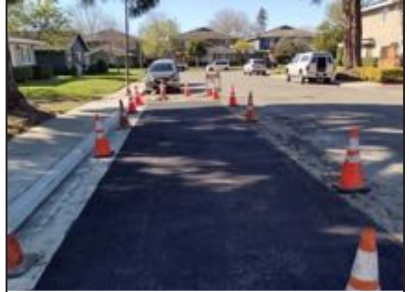
Diamond Street road rehabilitation (before & after), City of Capitola
