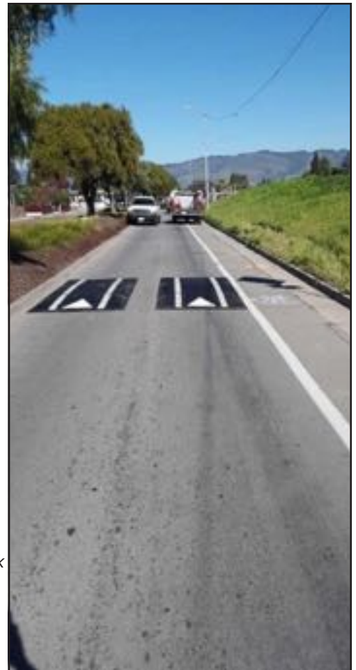
Speed hump installation, City of Watsonville
