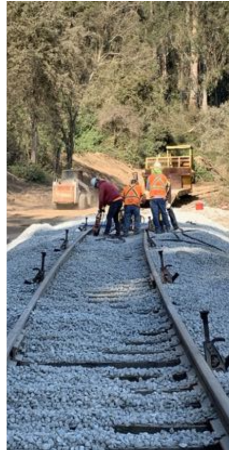
Crews work on storm damage repairs on the rail line.
