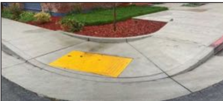
Left: Sidewalk replacement, City of Watsonville
