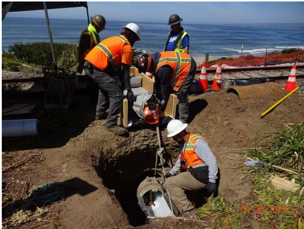
Figure 3 - Drainage culvert rehabilitation just south of the La Selva trestle
