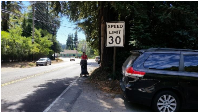
Photos 3 and 4: SB Highway 9 at PM 9.66 (less than 2 feet of walking space between the tree and edge line; scarred tree after head-on crash involving a heavy truck that destroyed the sign as well)
